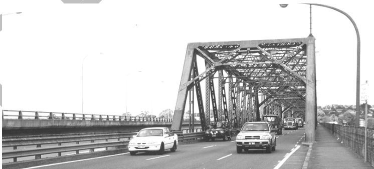
Fig. 1.3: Cars exiting the northern end of Tom Ugly's Bridge over the Georges River (NSW). It utilises a truss style beam while the new bridge alongside uses box girder construction.
