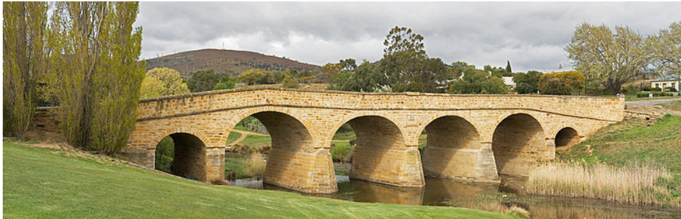
Fig 1.4: The Richmond Bridge in Tasmania is the oldest bridge in Australia; it is a sandstone arch bridge. ( http://en.wikipedia.org/wiki/File:Richmond_Bridge_Panorama_Restitch.jpg )
