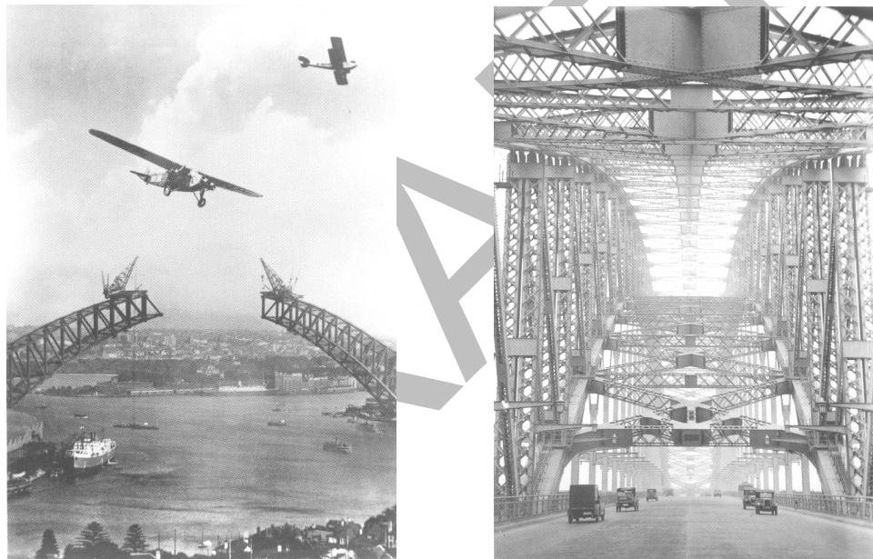
Fig 1.5: The Sydney Harbour Bridge; left, during construction and right, the day after the 1932 opening. (Photographs reproduced with permission, State Library of NSW).
