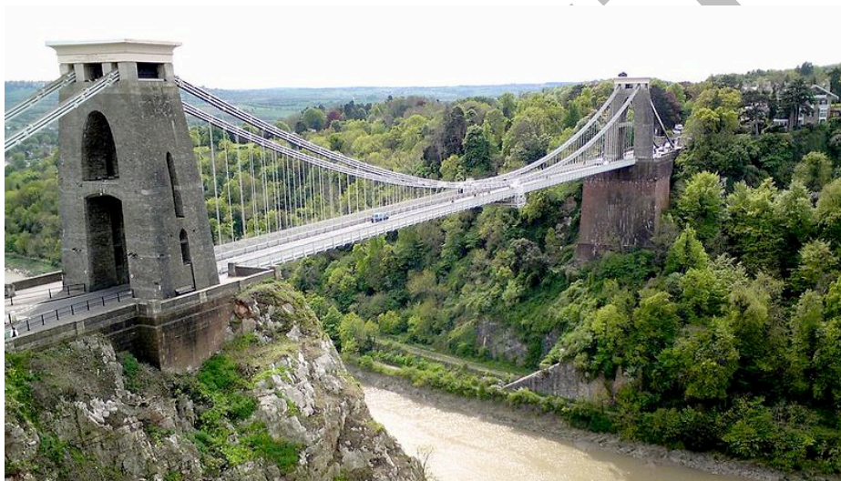
Fig. 1.7: Brunel's Clifton suspension bridge; the "chains" are made with wrought iron plates.
